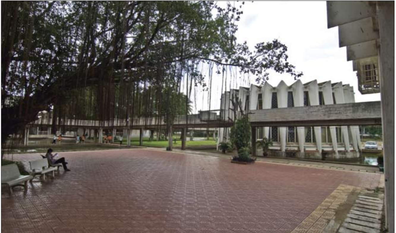
Institute of Foreign Languages: Long elevated walkway with the library in the background
